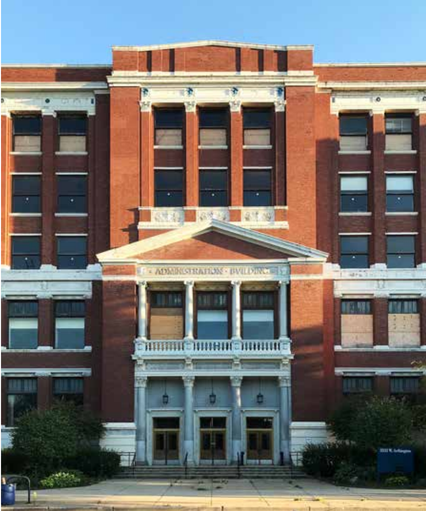
Close-up of Sears Administration Building main entrance.
