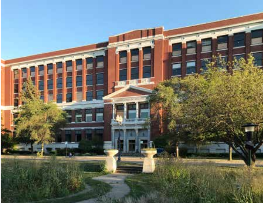
Sears Administration Building, view looking southeast across W. Arthington Street.
