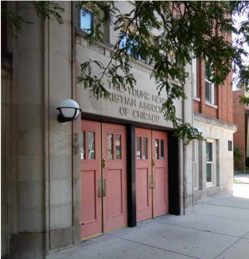
Close-up of Wabash Avenue YMCA main entrance.
